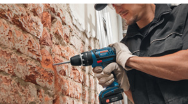
Phase 2 – Interior fitting
